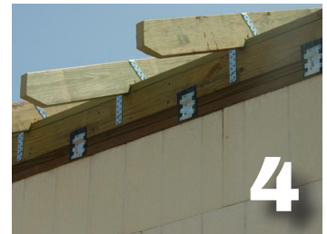
1) Hurricane brace; 2) Metal roofing; 3) Secondary water resistance; 4) Roof framing (Photos courtesy of LaHouse Research & Education Center )
