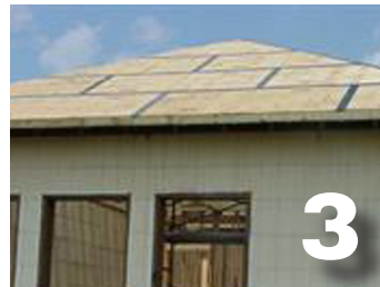
1) Hurricane brace; 2) Metal roofing; 3) Secondary water resistance; 4) Roof framing (Photos courtesy of LaHouse Research & Education Center )
